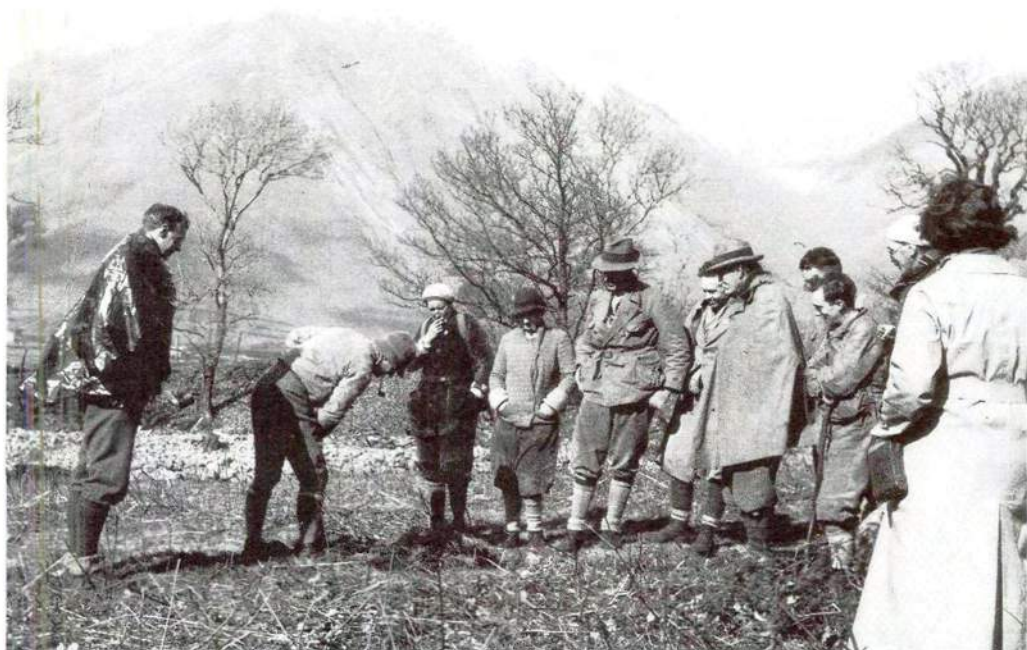
Cutting the First Sod at Brackenclose, 13 April, 1936
